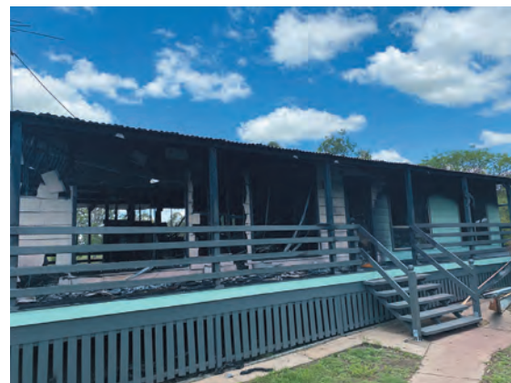
The owner of this property was left with nothing. The pack supplied by Gatton police allowed her to have a shower and clean away the pungent smell of smoke.
